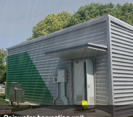
Rainwater harvesting unit at Intersurgical China
